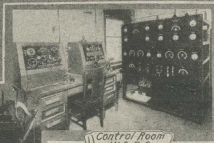
Control Room WSBC
